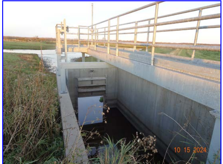
Photo 1 - Southwest Outlet structure.
