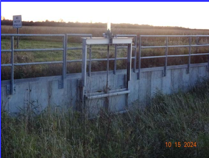
Photo 13 - Northeast inlet structure: Lateral gate connecting to the southern ditch.
