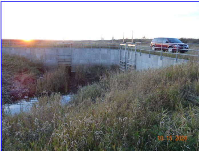
Photo 4 - Southeast control structure.
