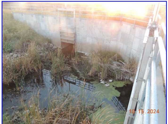
Photo 3 - Southeast control structure.
