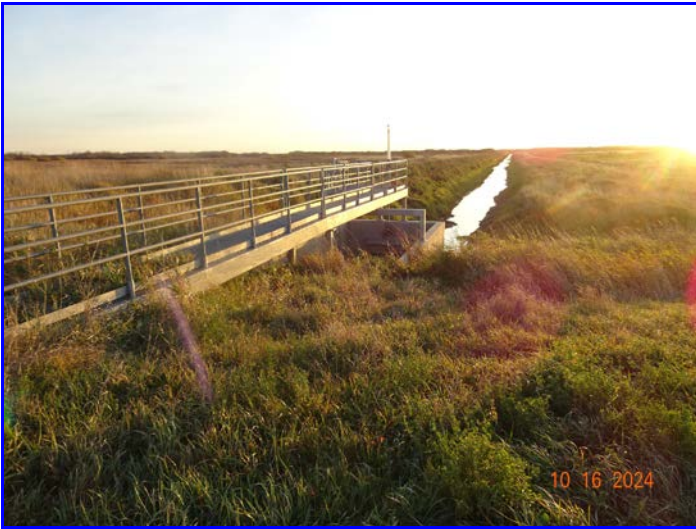
Photo 5 - West central control structure.
