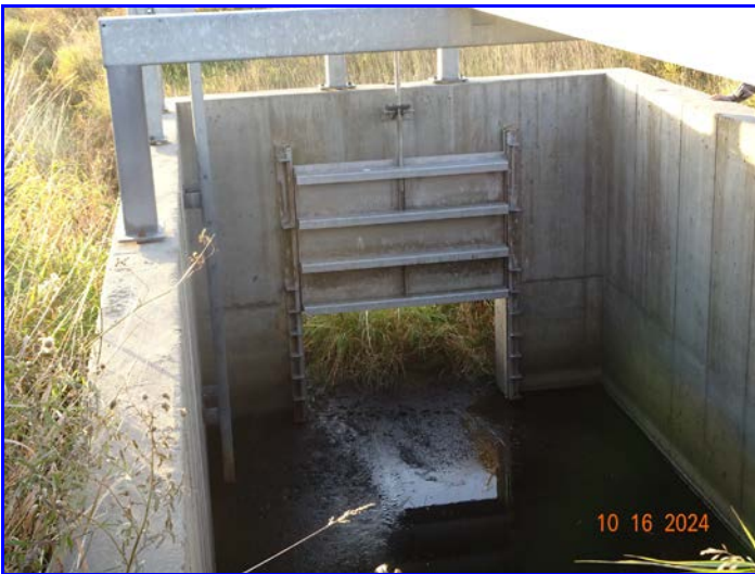
Photo 7 - Northwest Control Structure.
