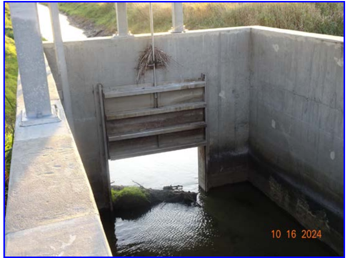
Photo 6 - West central control structure.
