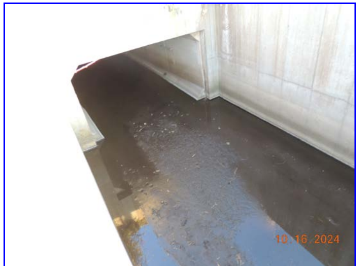
Photo 10 - Northwest stilling basin.
