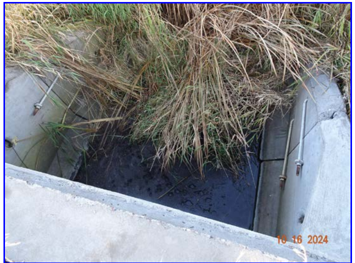
Photo 8 - Northwest conduit outlet.
