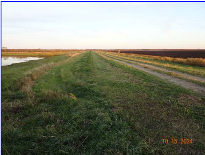
Photo 2 - Looking east down the southern embankment dam.
